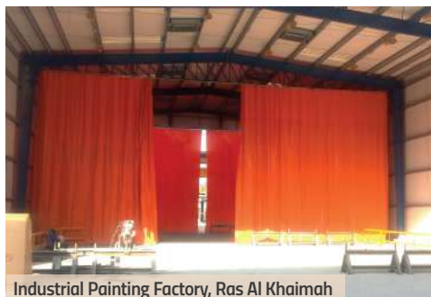
Industrial Painting Factory, Ras Al Khaimah
